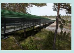
as possible, an 8.7-km-long conveyor belt will be built from Bunge to Storugns. The belt will mostly be covered, which will reduce both noise and dust emissions. It will also be raised to permit free passage by people and wildlife alike.
