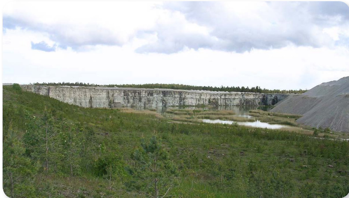
In the Klinthagen quarry on Gotland landscaping is going on in disused parts while quarrying proceeds in other parts of the quarry. This means that steep slopes are flattened and vegetation is planted. Some of the slopes are kept as they are because they represent typical natural landscape on Gotland. The water that collects on the bottom of the quarry has turned into a small lake frequented by birds.
